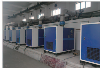
Shanghai Huaxin WWTP
