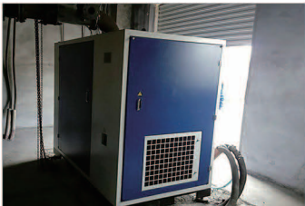
Shanshui cement plant
