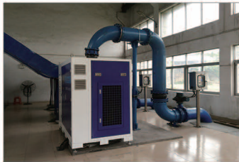
Shunde Lunjiao WWTP
